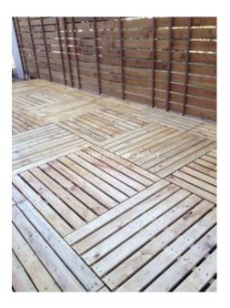
The easiest floor to put down is using pallets. You'll need to get several pallets; depending on the intended size of your storage shed. The pallets should rest on the breeze blocks and you'll have to fill in the gaps in the wood. You want a solid floor!
