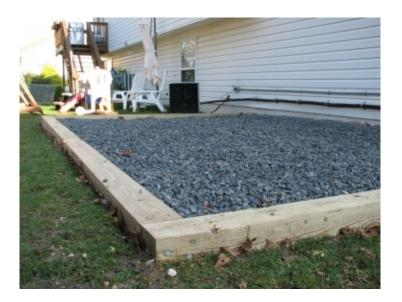
The first step must be to complete the base. It is best to create a shed on a hard surface. This will prevent the damp from the soil rotting your wood.
