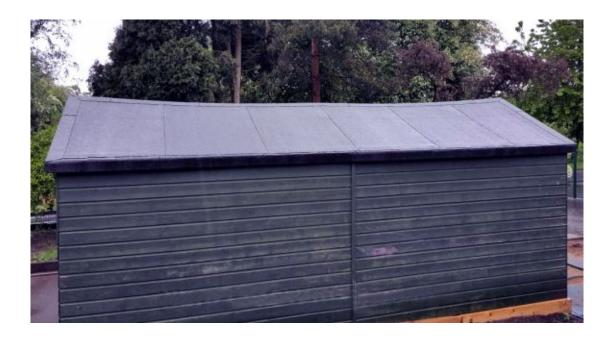
The roof can be fitted directly onto the top level of wood. It is easiest to use roofing felt although tarpaulin can be used if necessary.
